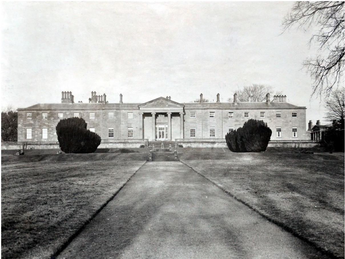
South Façade at Hillsborough Castle, circa 1926
