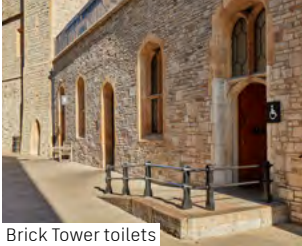
Brick Tower toilets
